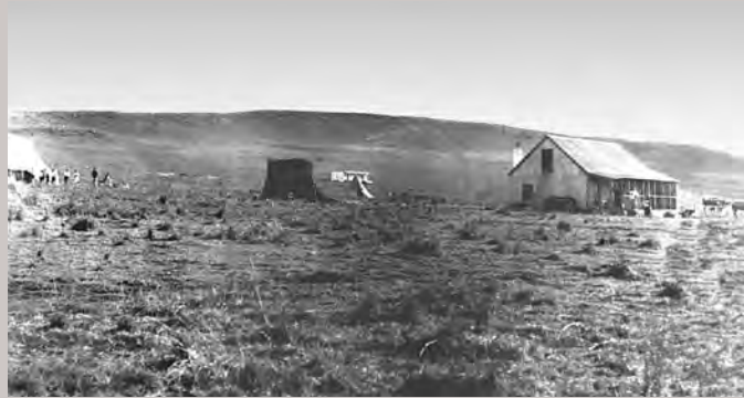
Tolstoy Farm: main house, tent and the outhouses.
